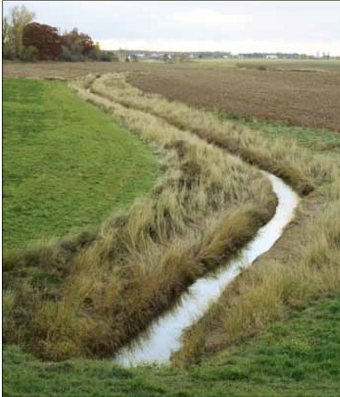
3-10 Drainage ditches allow water to drain from the fields and exit the dykelands.
